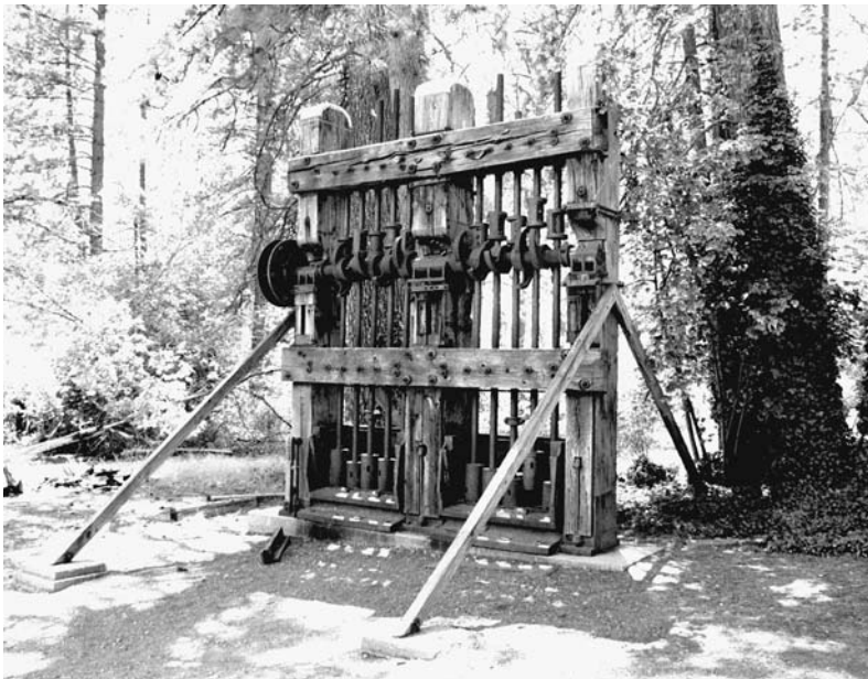
This ten-stamp mill at the Empire Mine near Grass Valley was used to crush gold ore into powder during the milling process. At its peak, the mill at the Empire Mine had 80 stamps that operated 24 hours a day and could be heard for miles.
