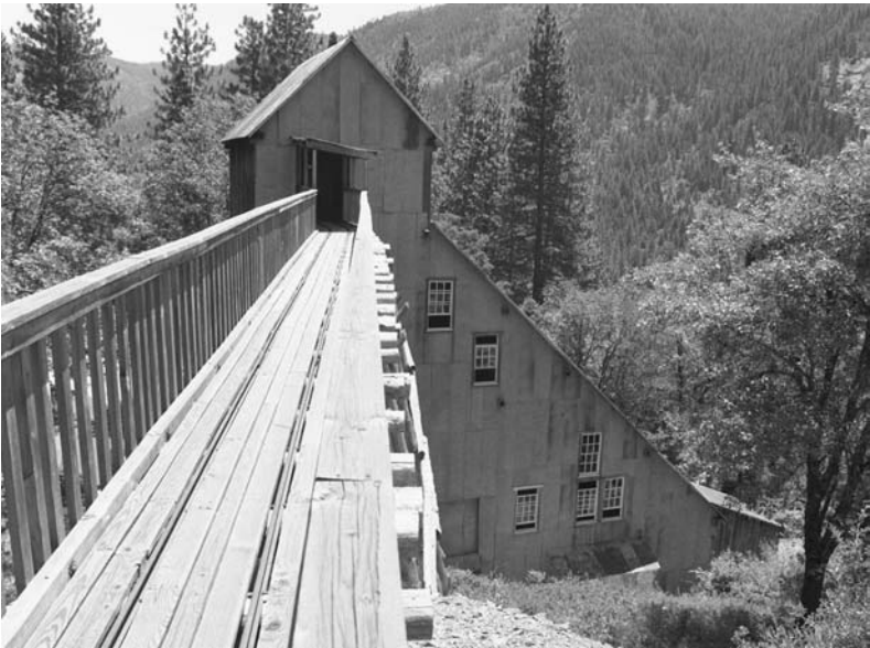
Gold ore from the Kentucky Mine was carried in small ore cars across this trestle to the mill where the gold was processed. The mill is open for tours and is typical of the mills of the Sierra Nevada gold belt.
