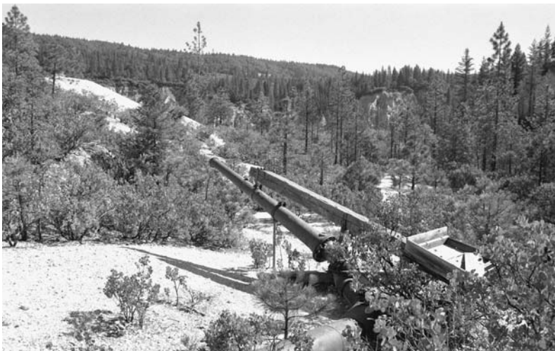
This monitor near the West Point Overlook now lies silent on the floor of the Malakoff Pit. During the 1870's as many as a dozen monitors were used in the hydraulic mining of the pit.
