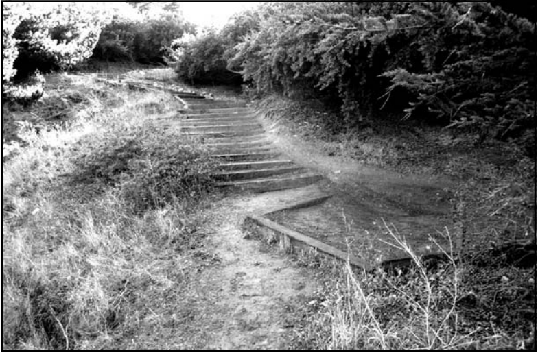
These steps go down the landslide at the end of El Camino del Mar. The landslide removed a several-hundred-foot section of El Camino del Mar. Pieces of the old asphalt road surface can be seen in the landslide debris near the base of the steps.
